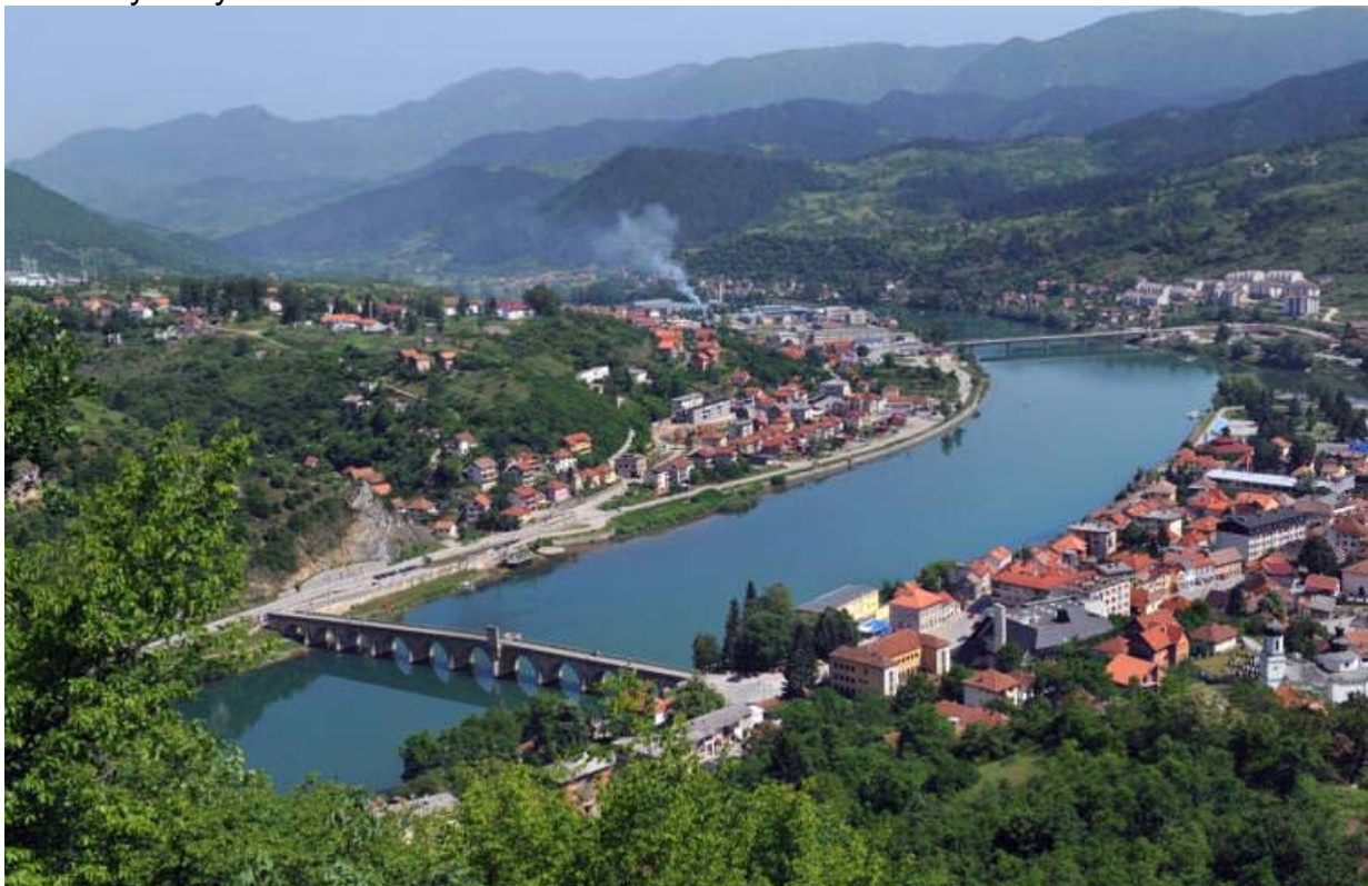
The Mehmet Paša Sokolović Bridge in Višegrad. Image by Bernd Zillich / Getty
